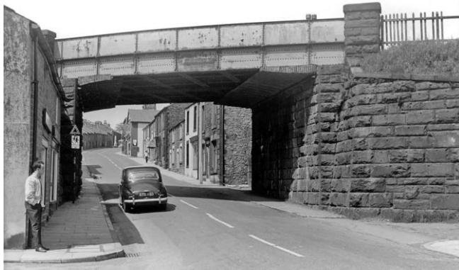
Photo 2. The old railway bridge crossing over School Lane, Brinscall
