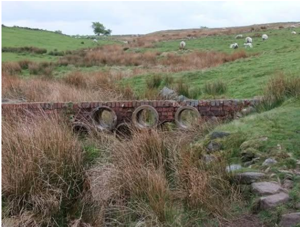
Photo 1. Remains of pipes from decoy post up on the moor
