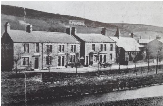
Photo 1. Quarry Road pre-1906 with the original Goit running between Brinscall and Withnell. The brick wall separating the Goit from Railway Rd can be seen at the bottom of the photo.
